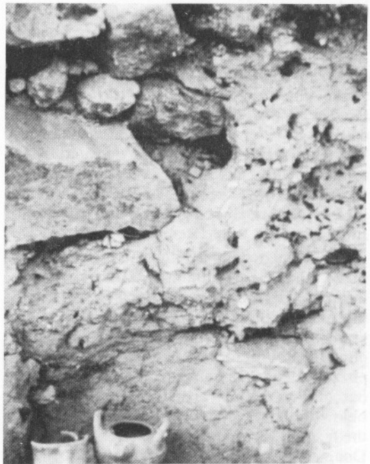
FIG. 1. Holes of nests of A. crinipes and O. latreillei in the walls of the archaeological buildings at Akrotiri, Santorini.
